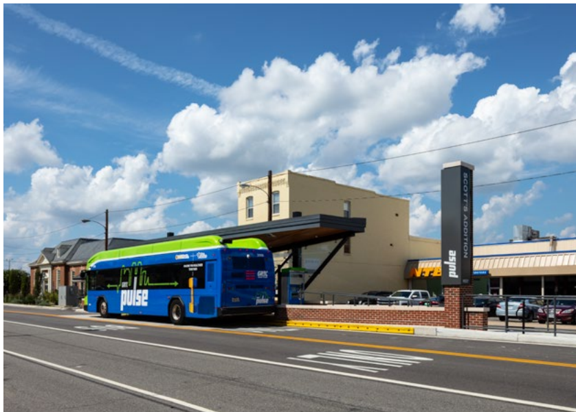
Images on this spread and on the cover: VDOT GRTC The Pulse BRT Design-Build, Richmond, VA
