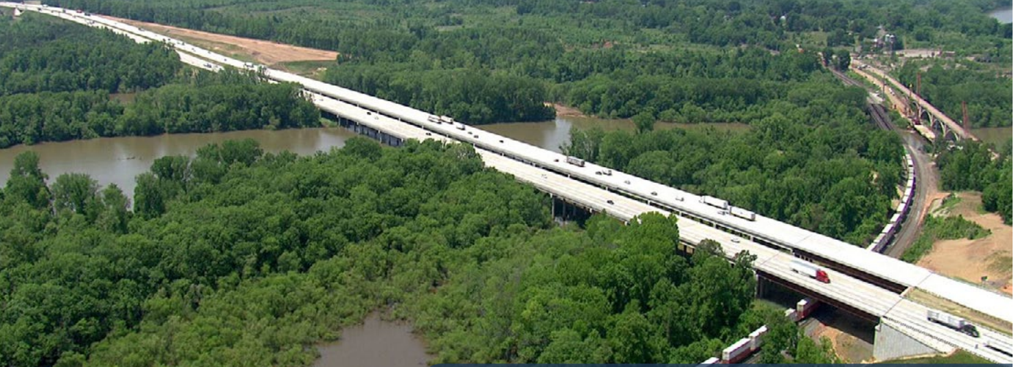
North Carolina DOT, I-85 over the Yadkin River Design-Build, Rowan and Davidson Counties, NC
