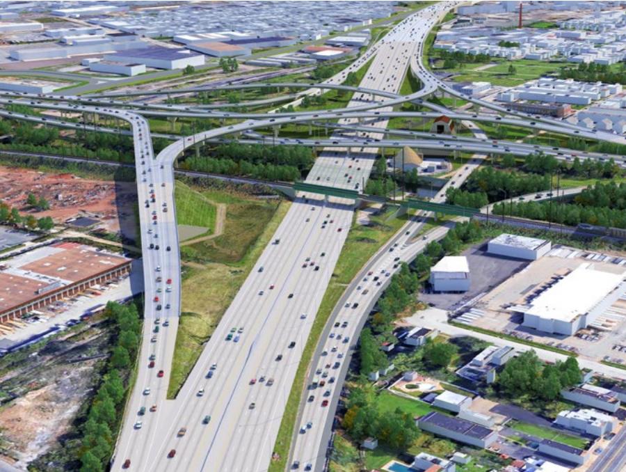
PennDOT, I-95 Section BRI – Betsy Ross Interchange Reconstruction, Philadelphia, PA
